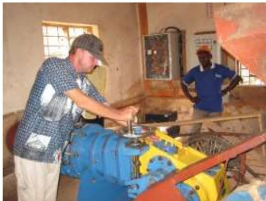
In the Hydro-Electric-Plant of **Kindimba**, which we supported since electrification, the power generation failed after lightning, destroyed the control unit. Bro. Maximilian has installed a new control unit, provided by Licht für Afrika so, that light has come back in time for Christmas.
